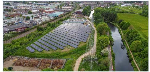
1.2 MWp of solar PV generation on old landfill, private wire to 2MW battery storage and Kempower Satellite DC charging System for eRCVs (installed by mer/Statkraft).
